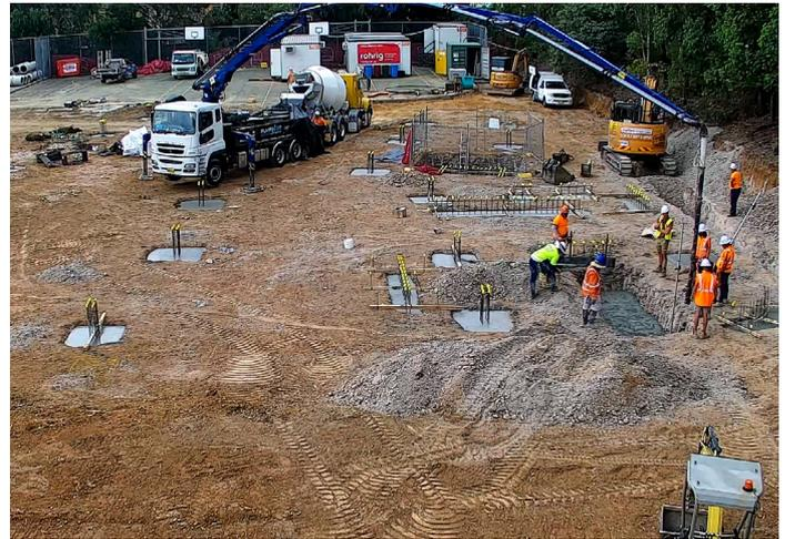
*All bulk excavation work has been completed and the detailed excavation work is near completion. The footings and major stormwater are at 80% completion and you will notice that vertical elements of the building now exist, with many of the ground floor columns now in place. The sewer connection has been established.*
