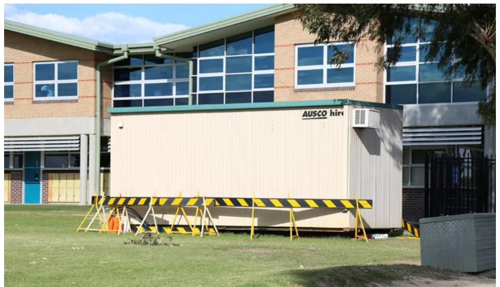
Service building located at the western, Morris Grove side of the green space closest to the long jump pits.
