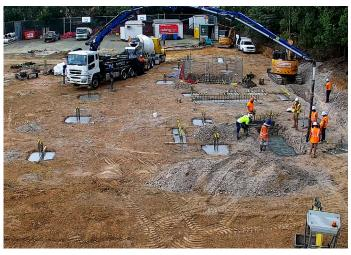
All bulk excavation work has been completed and the detailed excavation work is near completion. The footings and major stormwater are at 80% completion and you will notice that vertical elements of the building now exist, with many of the ground floor columns now in place. The sewer connection has been established.
