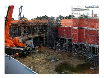
By the end of the first week of August, we would expect that the remaining vertical elements on the top floor will be completed. This includes the last concrete columns and the remainder of the structural steel on the top level. Internally, most of the formwork will be stripped out. Externally, work for housing the Kingspan external cladding will also be completed by that time.
