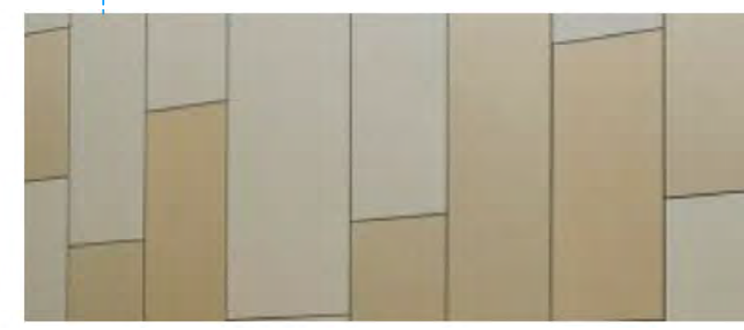
CFC panels colour matched to profiled metal facades
