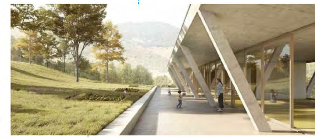
Angled concrete columns
