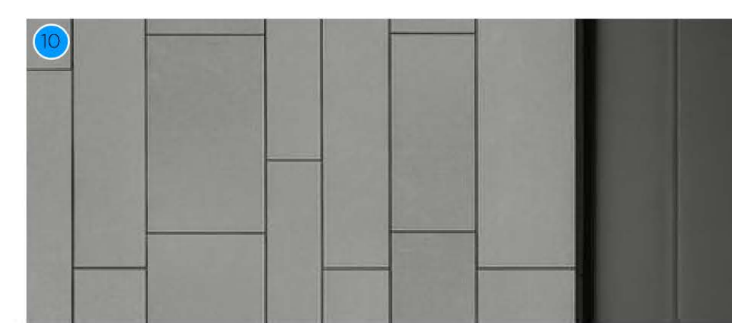
10. FC Cladding behind screened facade
