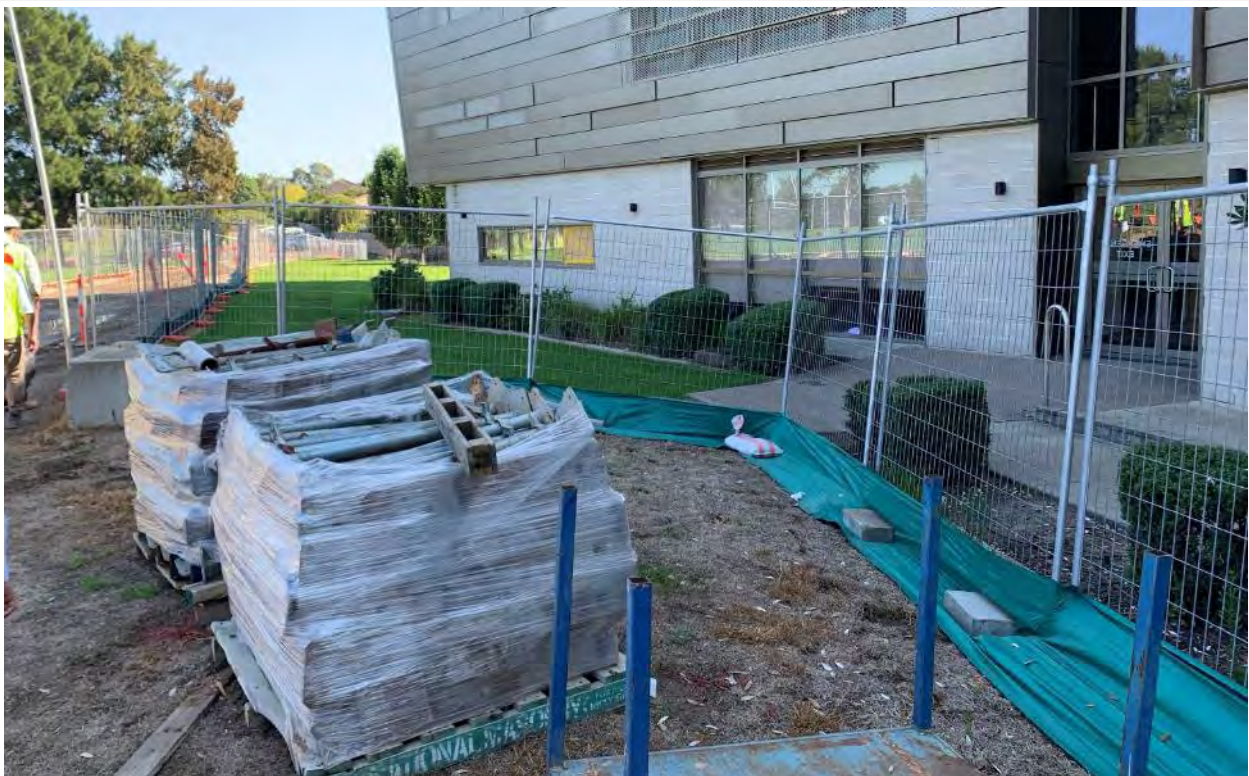
Sediment fence installed along the site boundary throughout the site. Designated areas for material storage.
