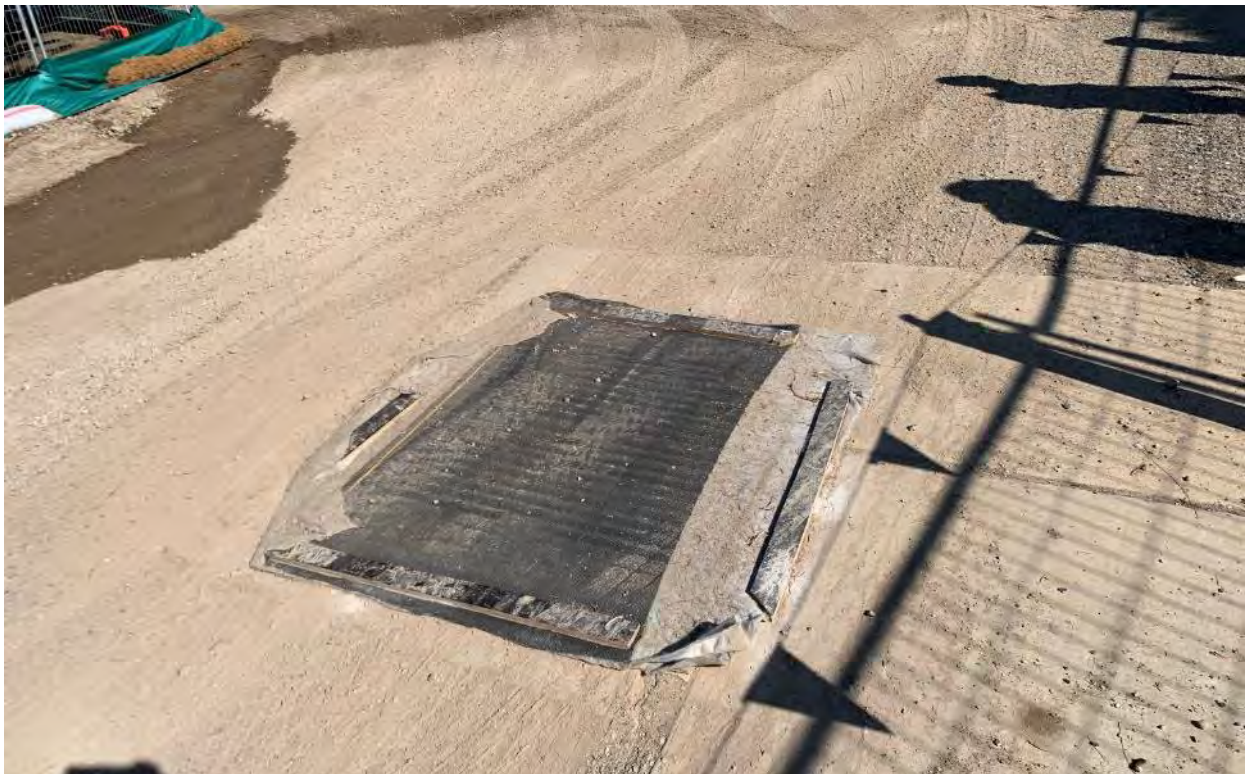
Pit drain fully covered with geofab.
