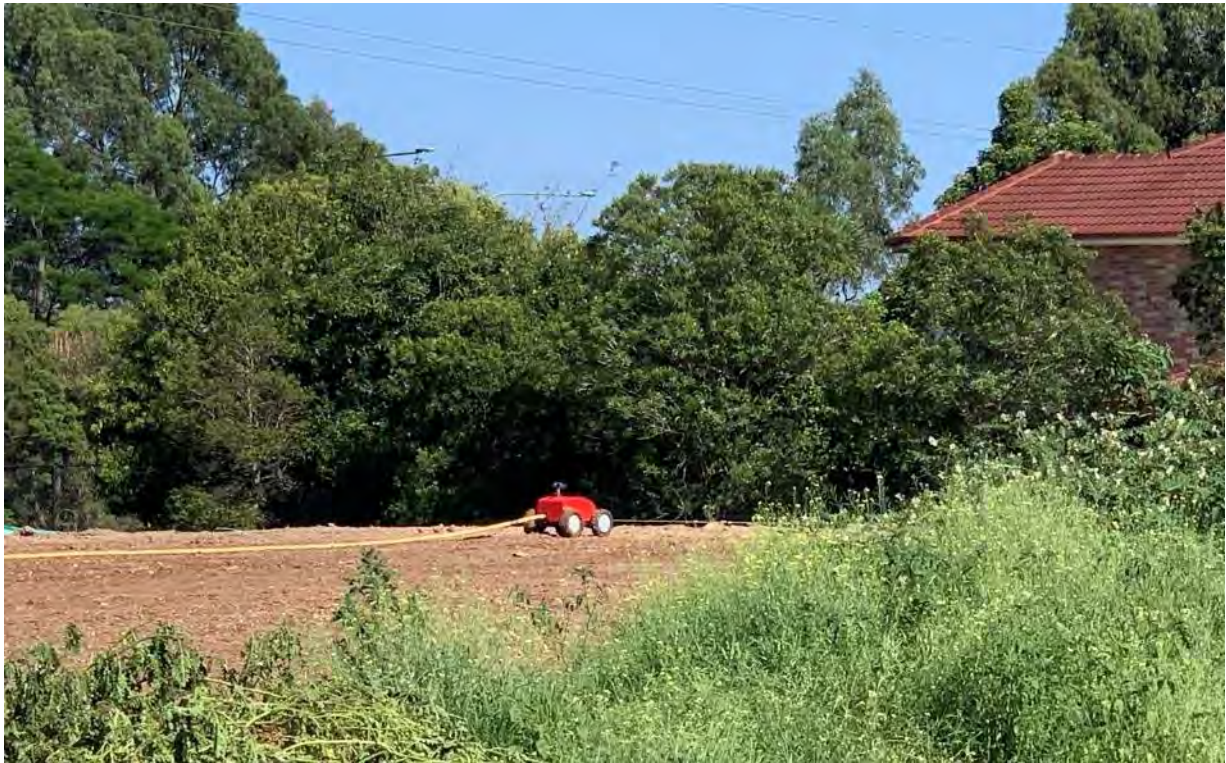
Irrigation sprinkler in place for dust suppression and soil stabilisation on stockpile area.
