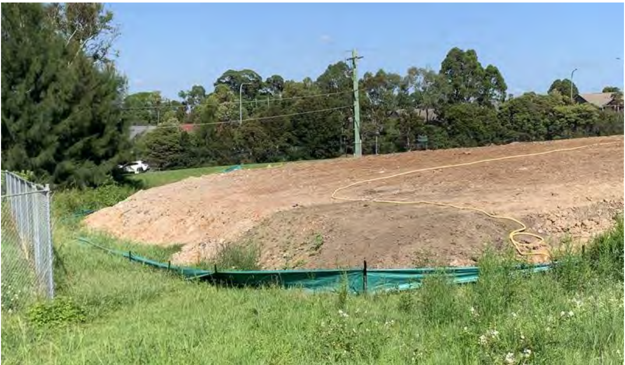
Sediment fence installed around nominated stockpile area and aligned to the erosion and sediment control plan.
