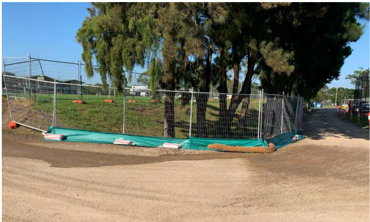
Sediment fence installed with sandbags and coir logs along the ATF fence at the site entrance.
