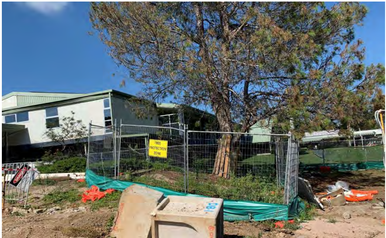
Tree Protection Zone established with a sediment fence installed around its perimeter.
