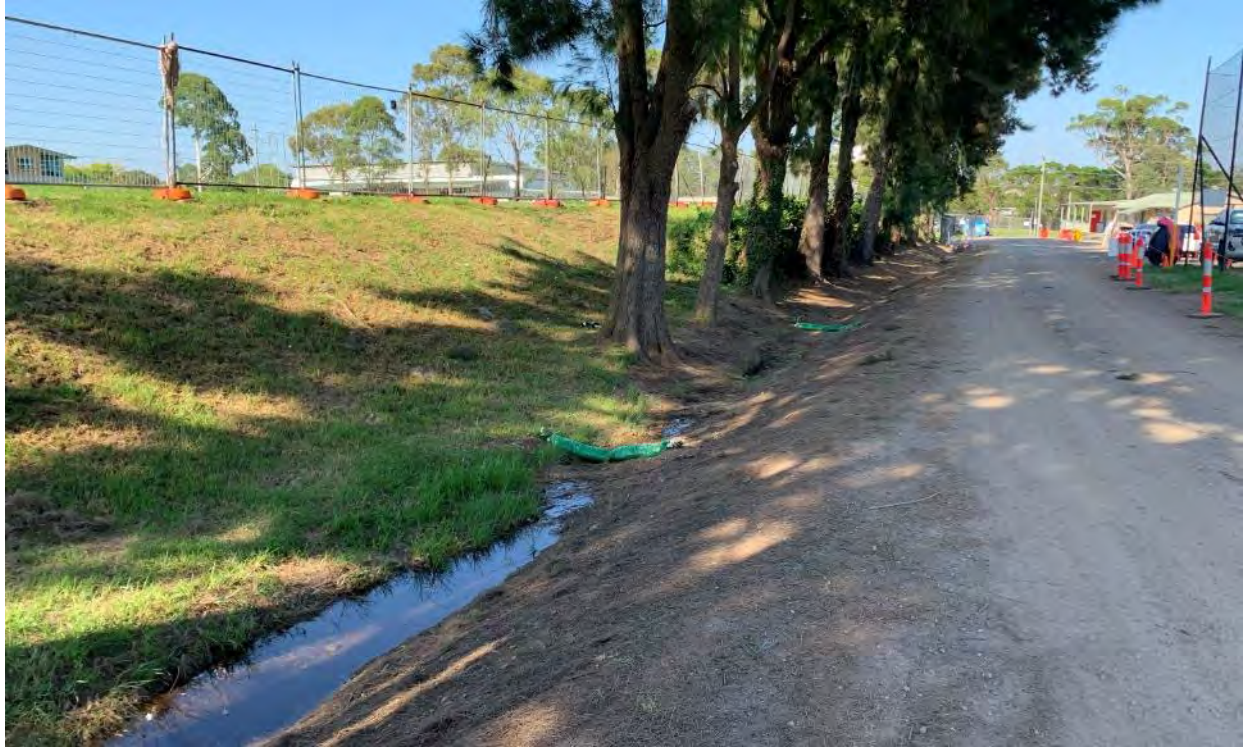
Sandbags placed along the swale drain leading to the WCC onsite dam managed by the school.
