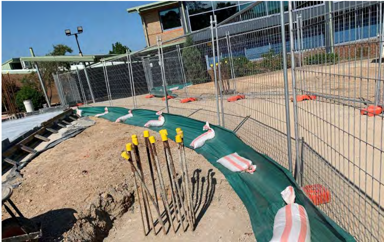
Sediment fence installed along the site boundary.
