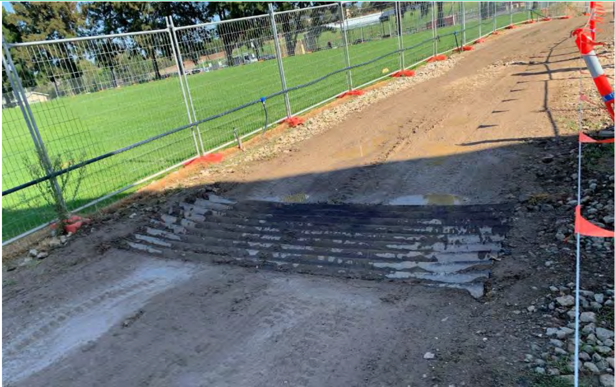
Rumble grid installed at the driveway.
