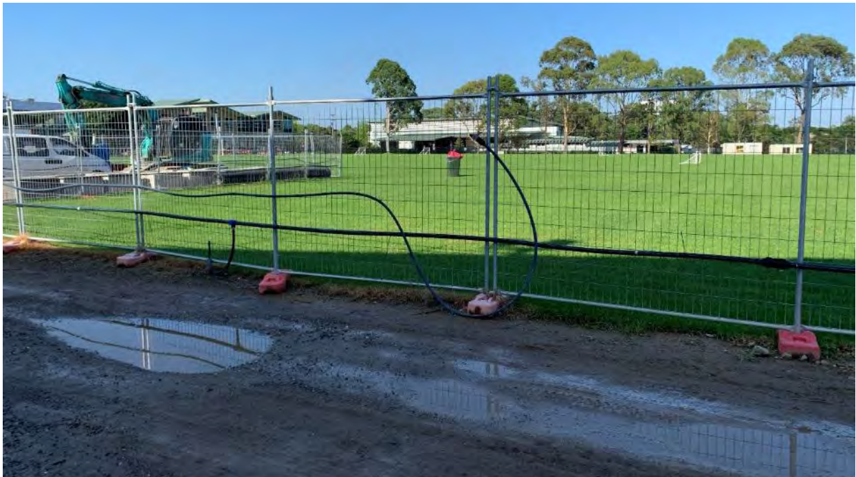
Sprinkler system installed along the driveway for dust suppression. Water pooled from rain the night before contained within the site boundary.
