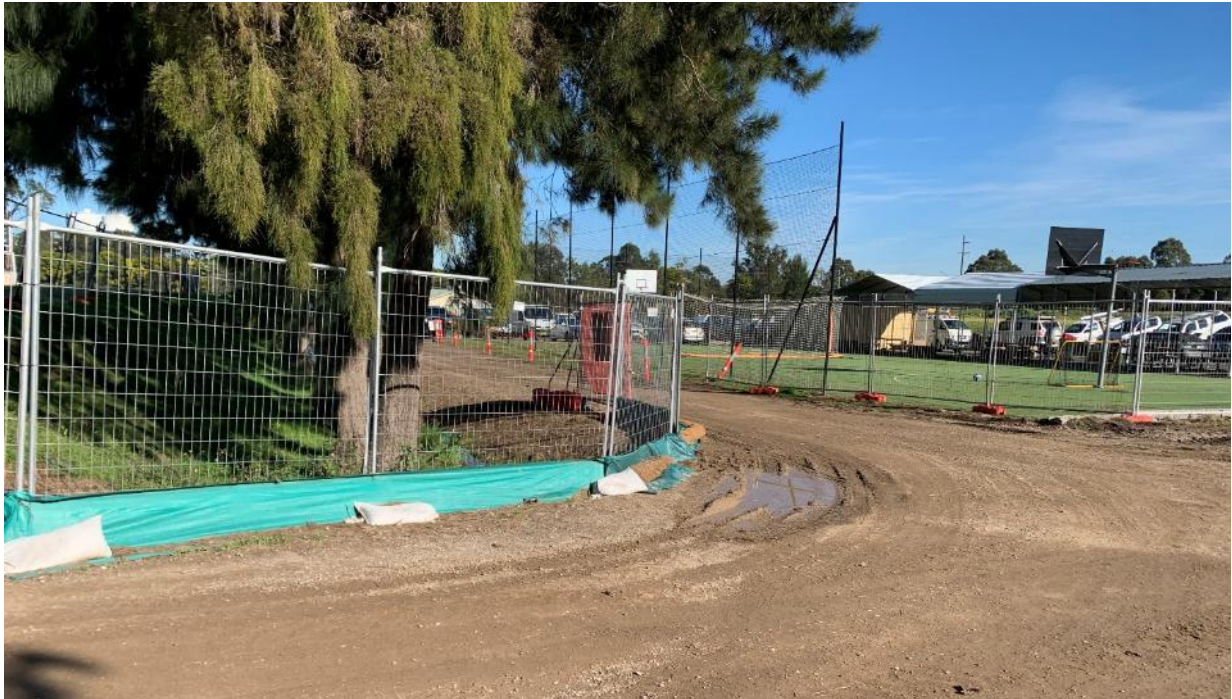
Sediment fence in place with sandbags and coir logs along the ATF fence at the site entrance.
