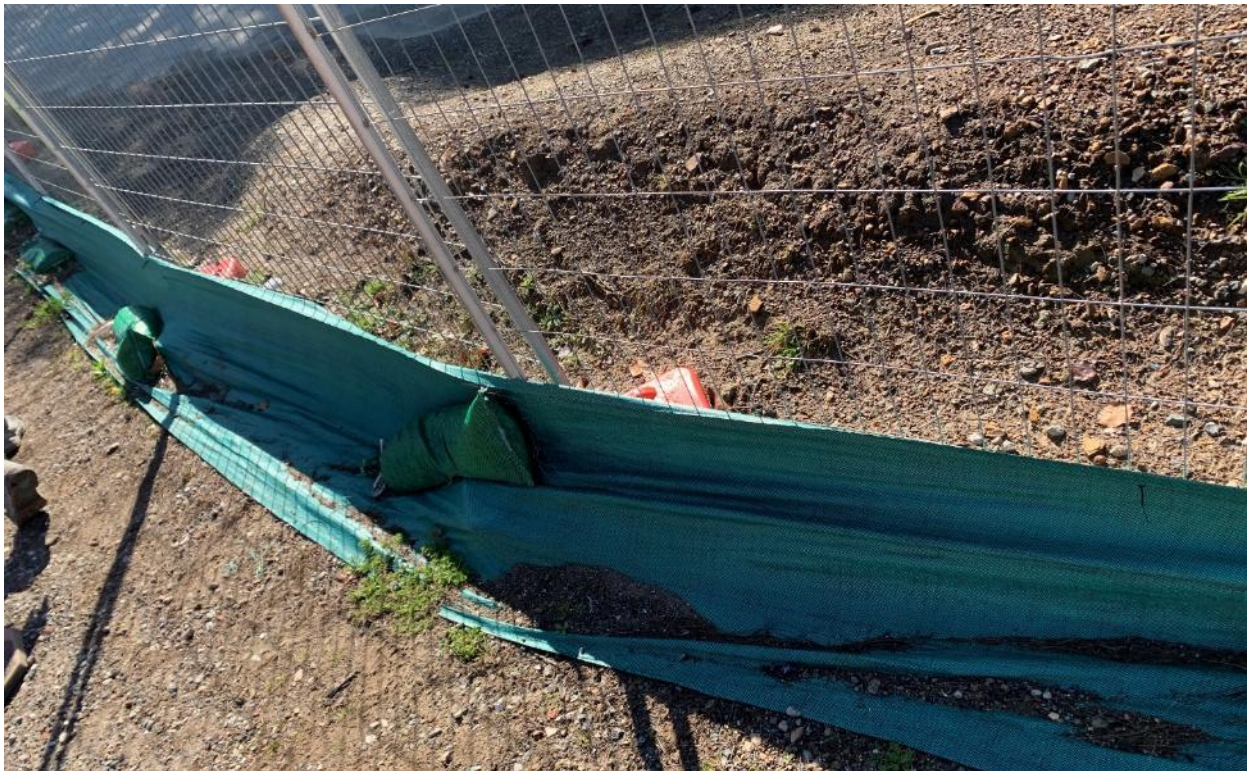
Sediment fence in place along the site boundary throughout the site
