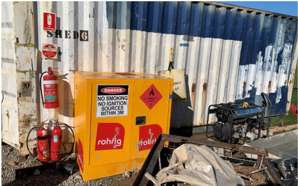
Chemical storage area with spill kit available.
