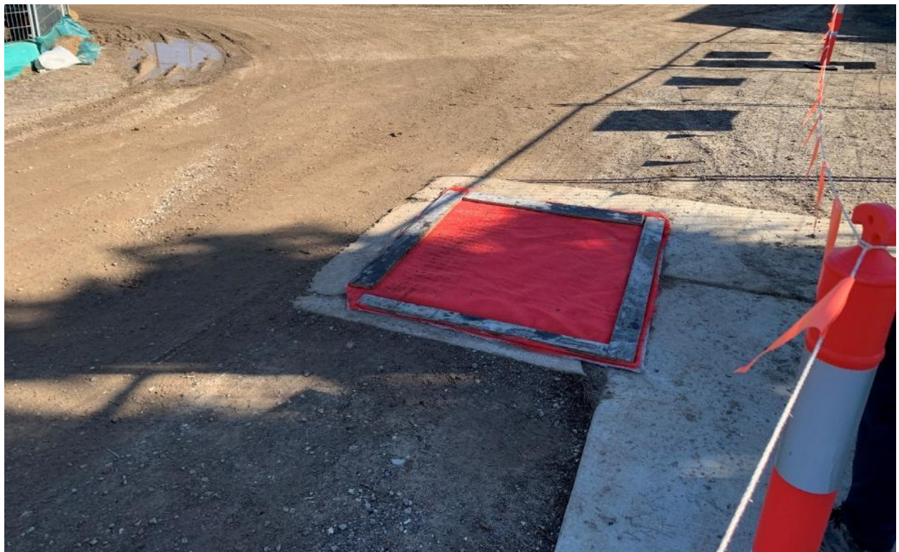
Pit drain fully covered with geofab.
