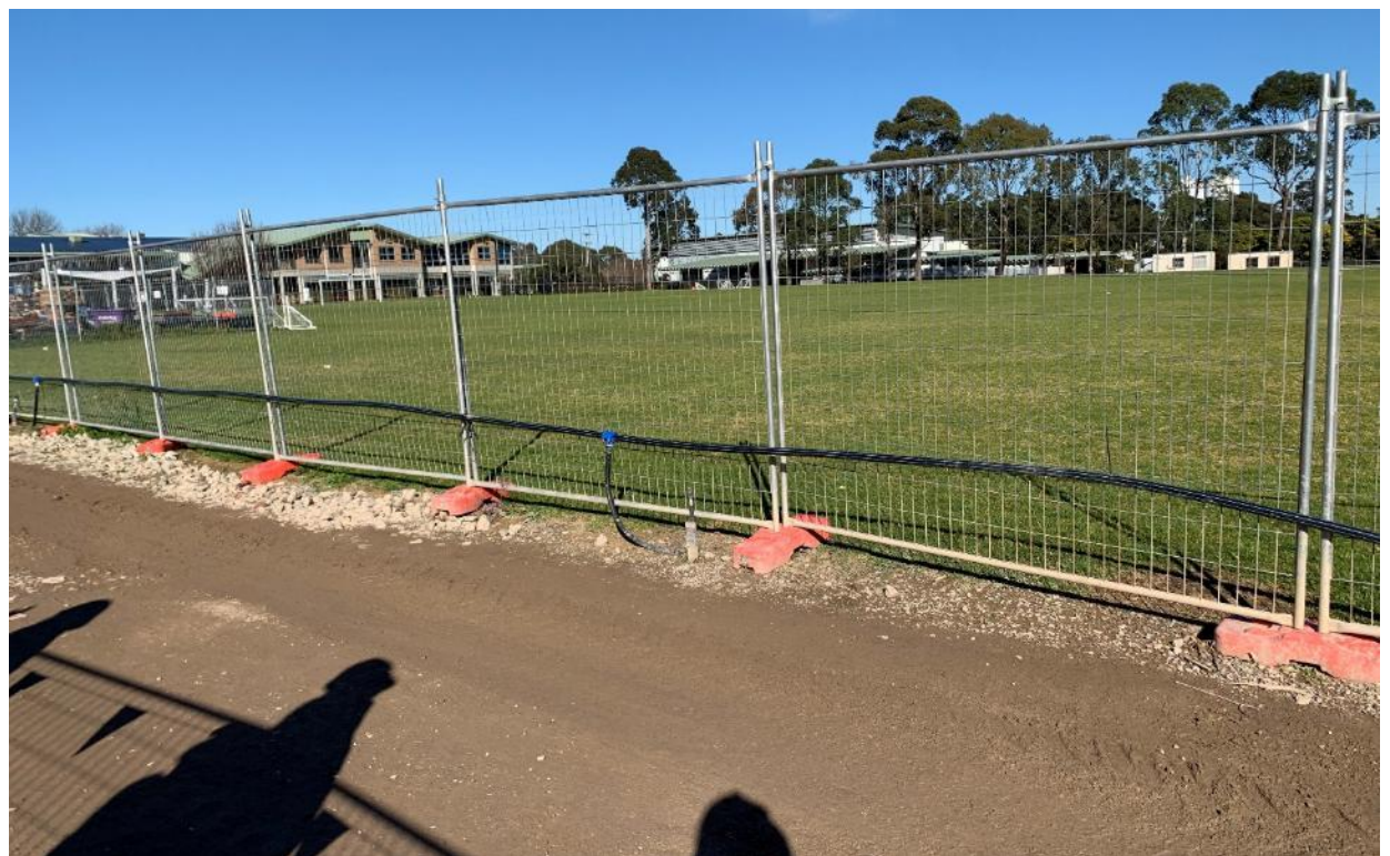
Sprinkler system installed along the driveway for dust suppression.
