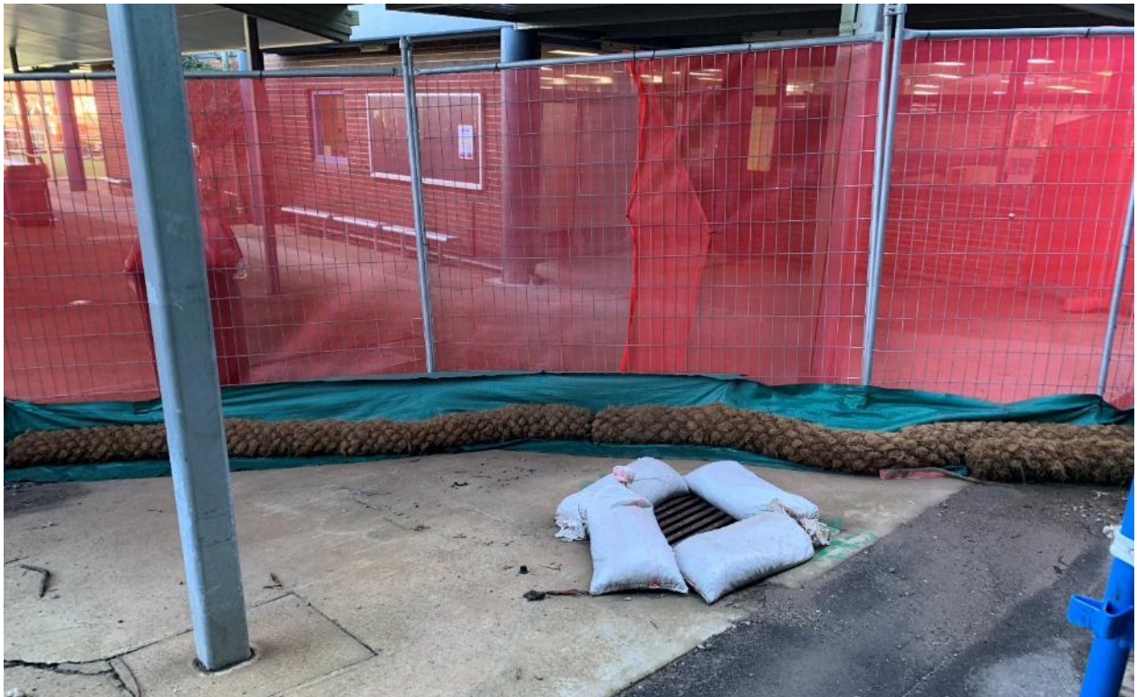
Sediment fence in place with coir logs along the ATF fence around the site boundary.
